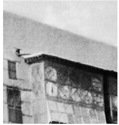
Solid rendered tall parapet
